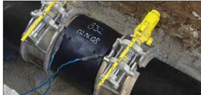
3.39 Re-rounding clamps for EF joints (source: +GF+)
